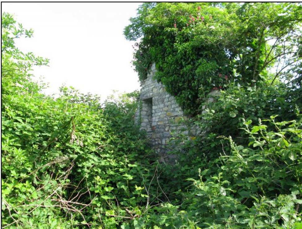
9. View from south-west of north-east end of ruined barn (probable dairy) to north-east of Lower Knowle Farm. Remains of walls of barn possibly survive beneath vegetation in foreground.
