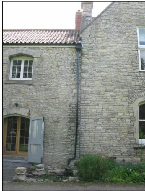
6. Detail of butting joint in façade. Most recent phase to left of image.
