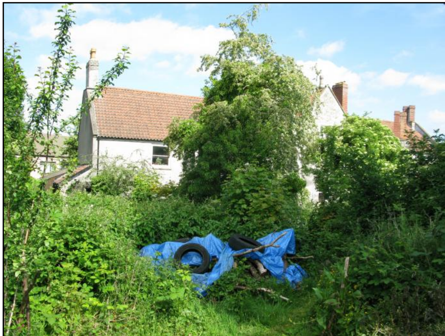
Frontispiece: Rear view of Lower Knowle Farm from south-east. Ruined dairy lies to right of frame, behind vegetation. Foundations of large barn lie just to left of image.
