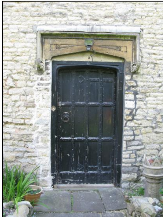
7. Detail of door in front (north-west facing) façade of Lower Knowle Farm, south-west end of building.
