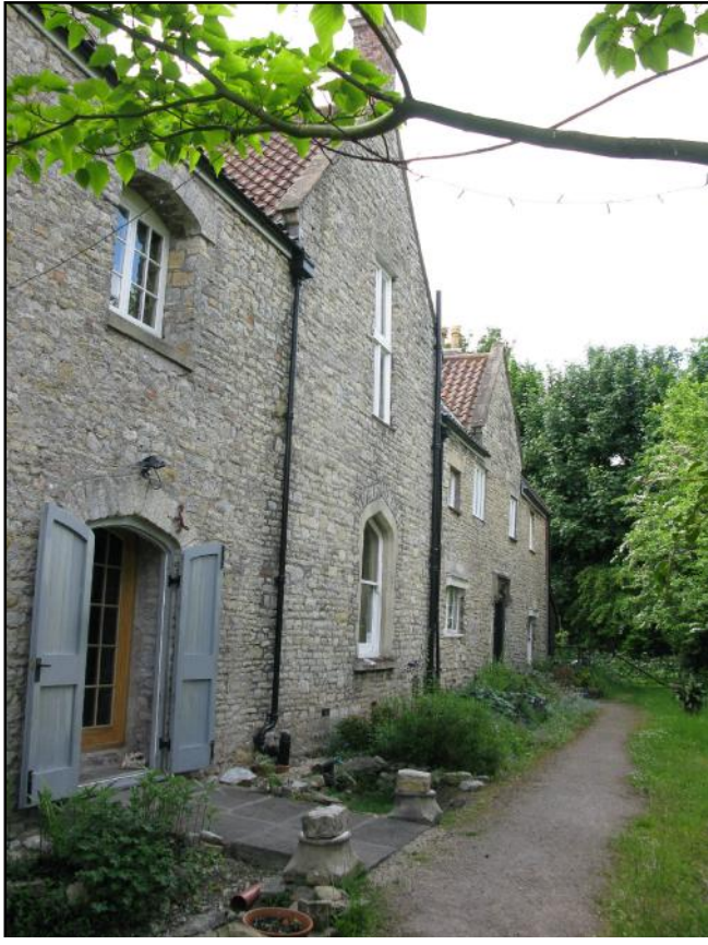
5. View from north of north-west facing façade of Lower Knowle Farm. Most recent phase to left of image.
